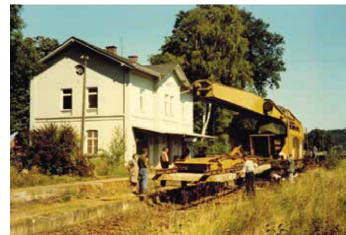
Schienenabbau in Mamming
